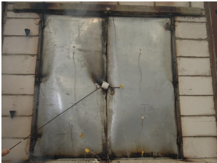
Fig. 6 – Unexposed Side after 107 Minutes
