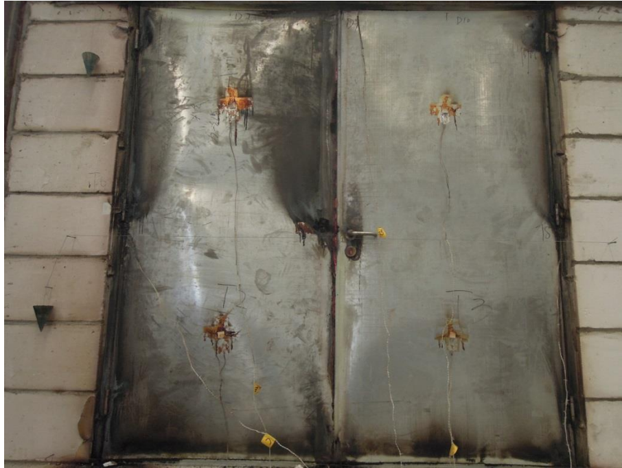
Fig. 7 – Unexposed Side after 150 Minutes
